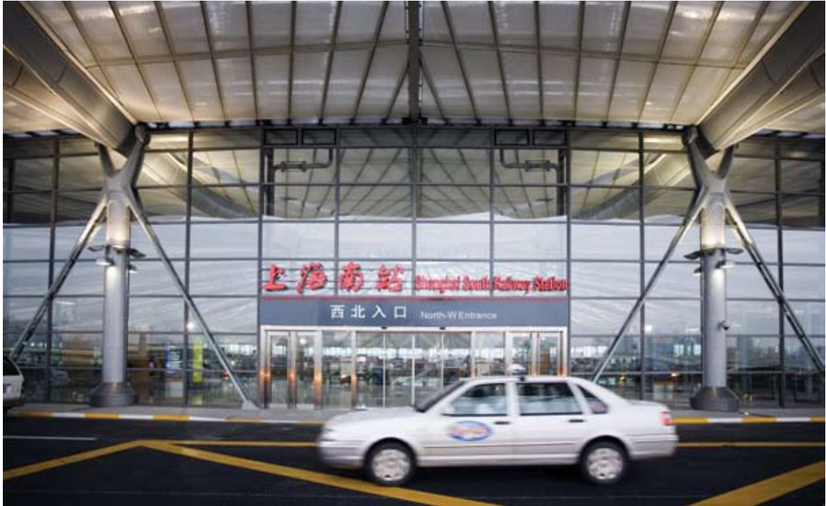
The roof's 15 m columns, of which there are 18, are closer to the center of the station. Its 9.8 m columns are farther from the center and form part of the facade, above. These shorter columns are reinforced by a bracing system comprising two ties 100 mm in diameter and are connected to the main roof beams using yokes of cast steel.
